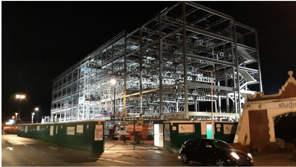
Teville Gate House Construction 12/12/2019
